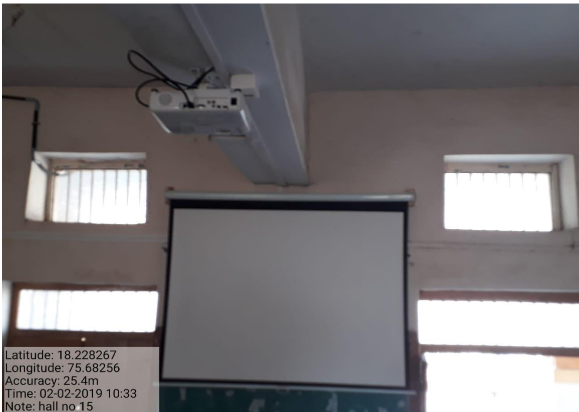
ICT Facility Hall No.15
