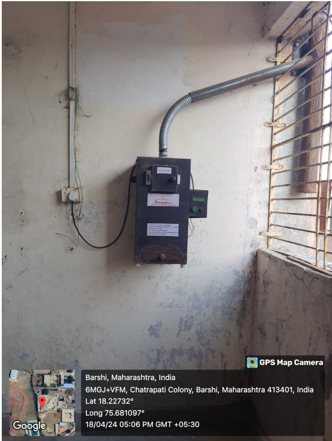
Disposable Machine of Sanitary Napkins on Ground Floor in Ladies Hostel
